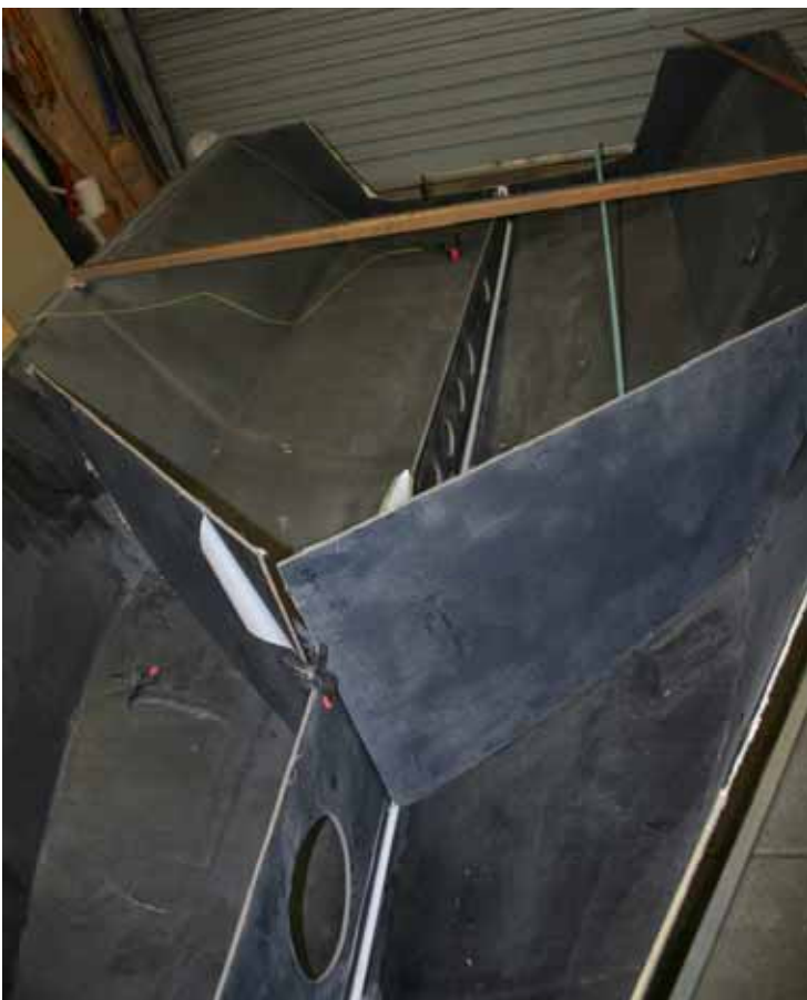
Below: Simon Blatchford's partly finished new hull with the bulkhead fitted and first longitudinal frame fitted and bonded. Flat panels make for easy construction. High res views one , two and three here.
